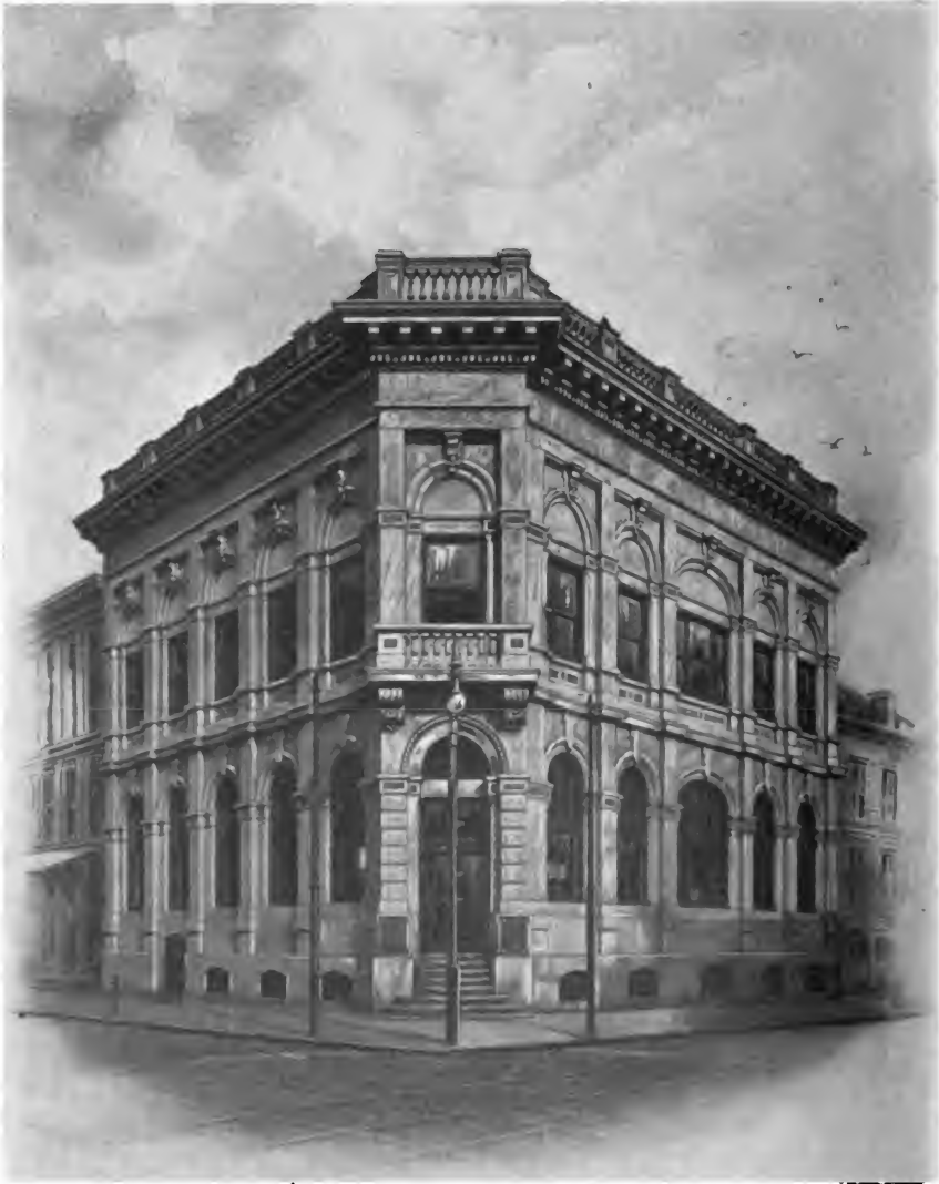
CITIZENS' NATIONAL BANK BUILDING, BALTIMORE.
